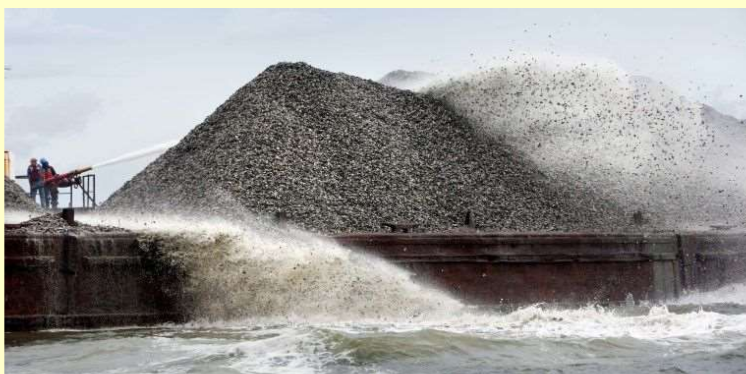
Water cannons used to spray fossilized shell on working oyster grounds on the James River. Harper, Scott . “Oysters' future rests on shells of ancient bivalves.” Norfolk Pilot, Jul 10, 2013.
