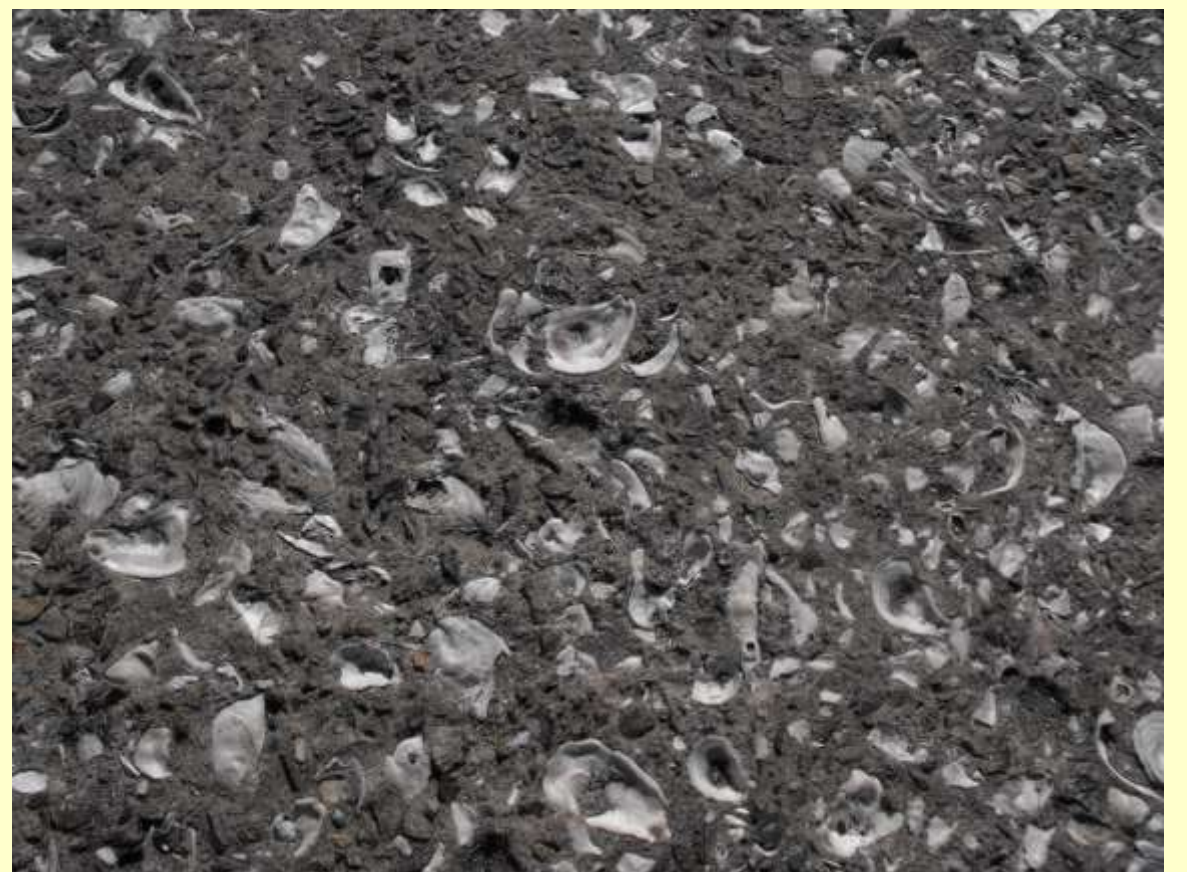
Example of tabby concrete walls made by the colonists from burning oyster shell which converts the calcium carbonate to quicklime. Shells were also used as aggregate. Wikimedia Commons.
